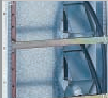
Cable connection compartment at the rear with one cable gland box per functional unit, internal separation Form 4 Type 7 acc. to BS EN 60439
